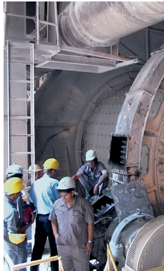
Inspection of a ball mill in a cement plant
