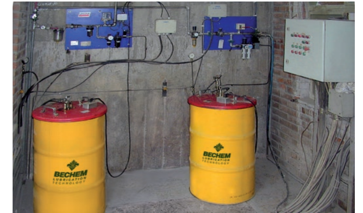
Drums of Berulit GA 2500 connected to spray systems
