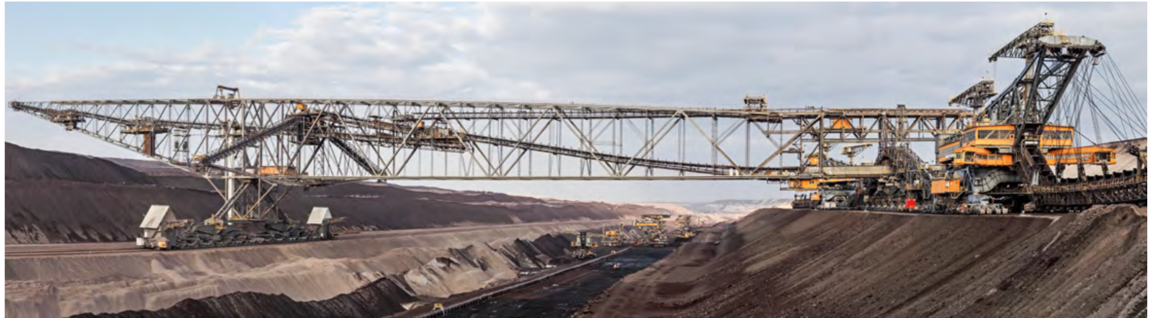
Overburden conveyor bridge in lignite open cast mining
