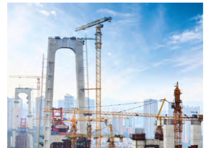
Crane in bridge construction
